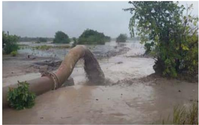
Fig.17: Tailings Discharge Column
