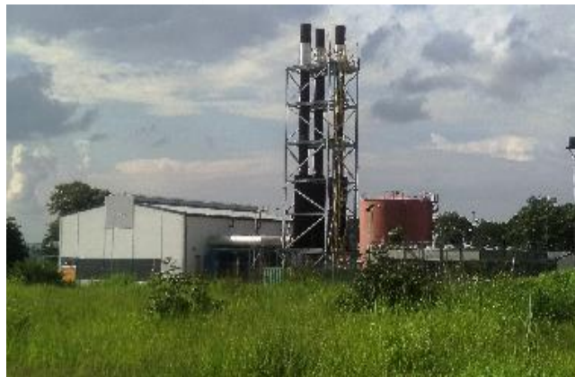
Fig.12: Diesel Generator Stacks
