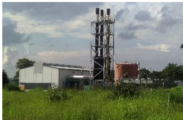
Fig.12: Diesel Generator Stacks
